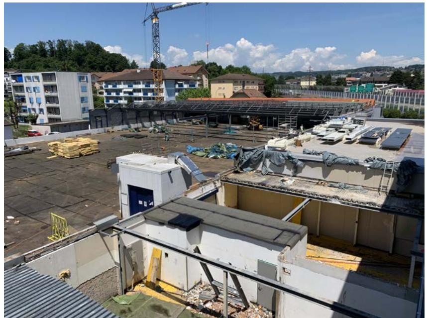
↑ Construction site of the Galaxis Lausanne-Ecublens distribution centre
