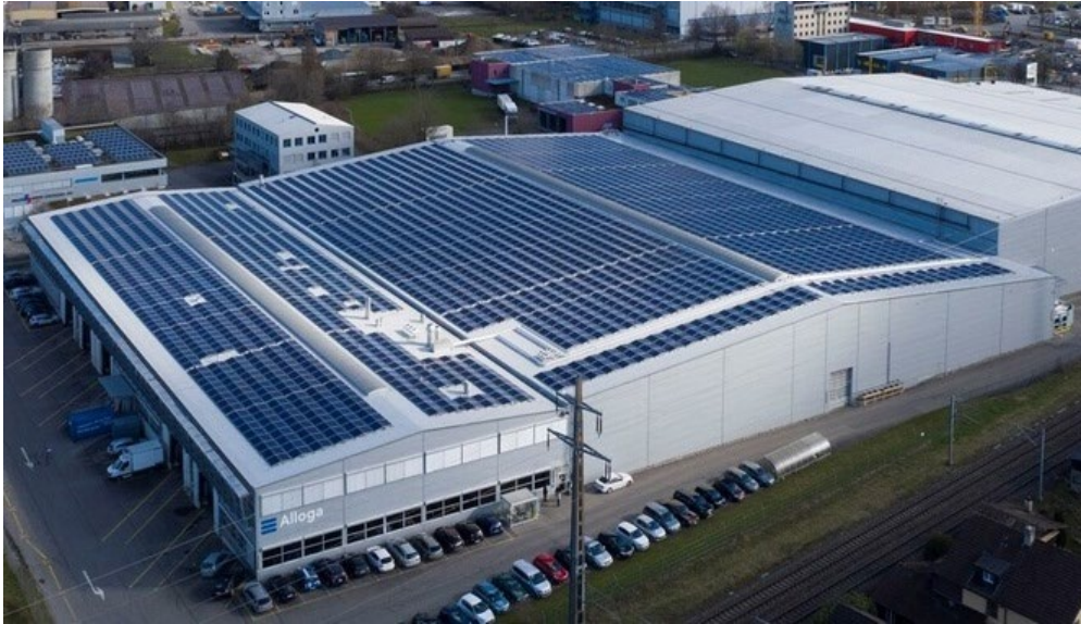
Solar panels on facilities in Burgdorf, Ecublens and Niederbipp
